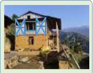
Mix structures are considered safe, if lower masonry structure is as per requirement. For upper structure, bracing or vertical props with proper connections shall be advisable if not provided.
