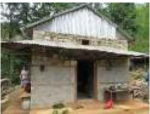
One+Attic by stone masonry in mud mortar with wooden band
