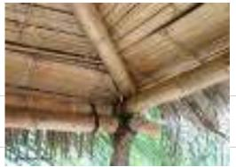
Vertical, Horizontal & Diagonal members connection using Lacing (Jute, Lylion, or equivalent) Techniques
