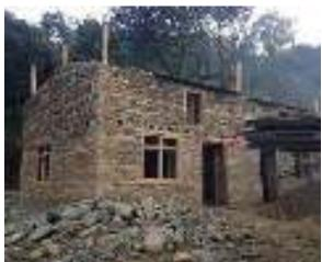
Two storeys constructed by stone masonry in mud mortar.
