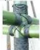
One Vertical, Two Horizontal members fitting connection combined with lashing technique
